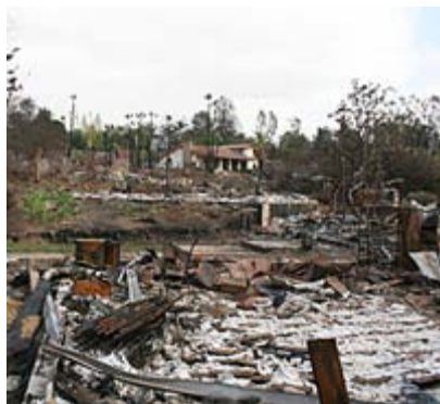
Ruins of two homes in The Trails community burned during the Witch and Guejito fires in 2007. (Photo Credit: NIST)
